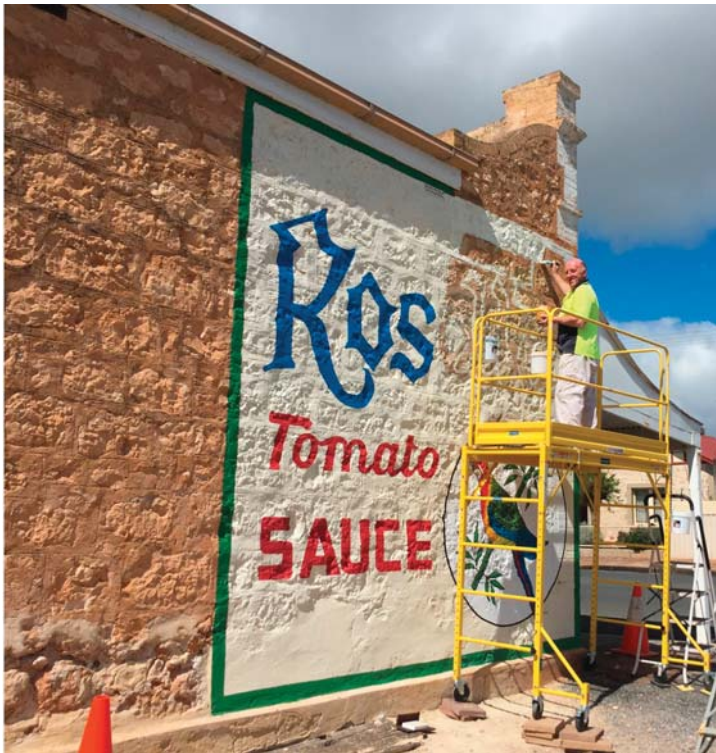
Rob Matthews helps on the scaffold doing 'filling in' for Julie.
